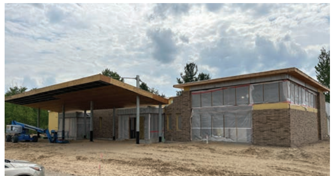
May 2024: Received brick delivery and began masonry work.
