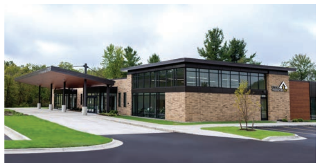
October 2024: Building was completed!
