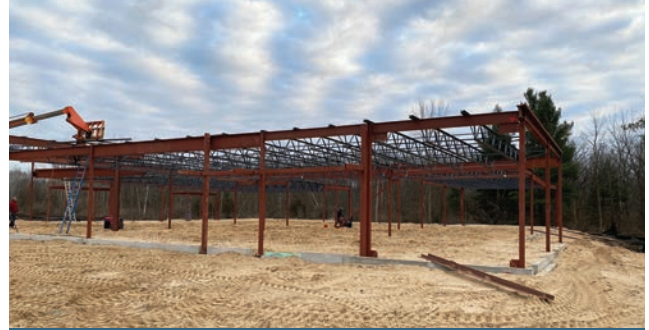
December 2023: Set structural columns and main support beams.
