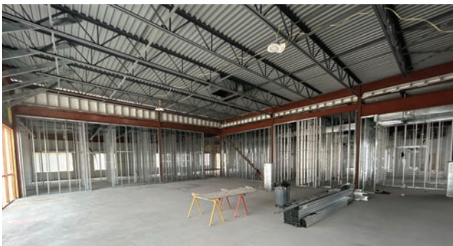
March 2024: Completed interior slab and interior wall framing.
